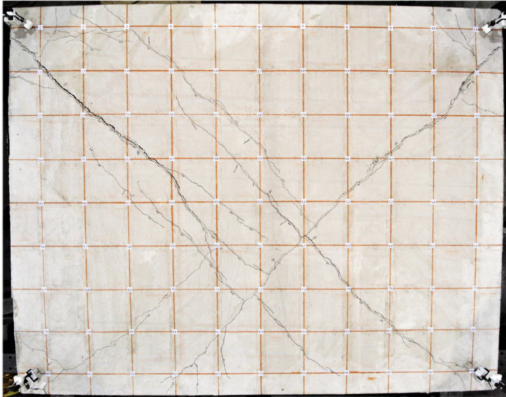
Figure 4.3 Diagonal Tension Cracking of Steel Deck-Slab Diaphragm
