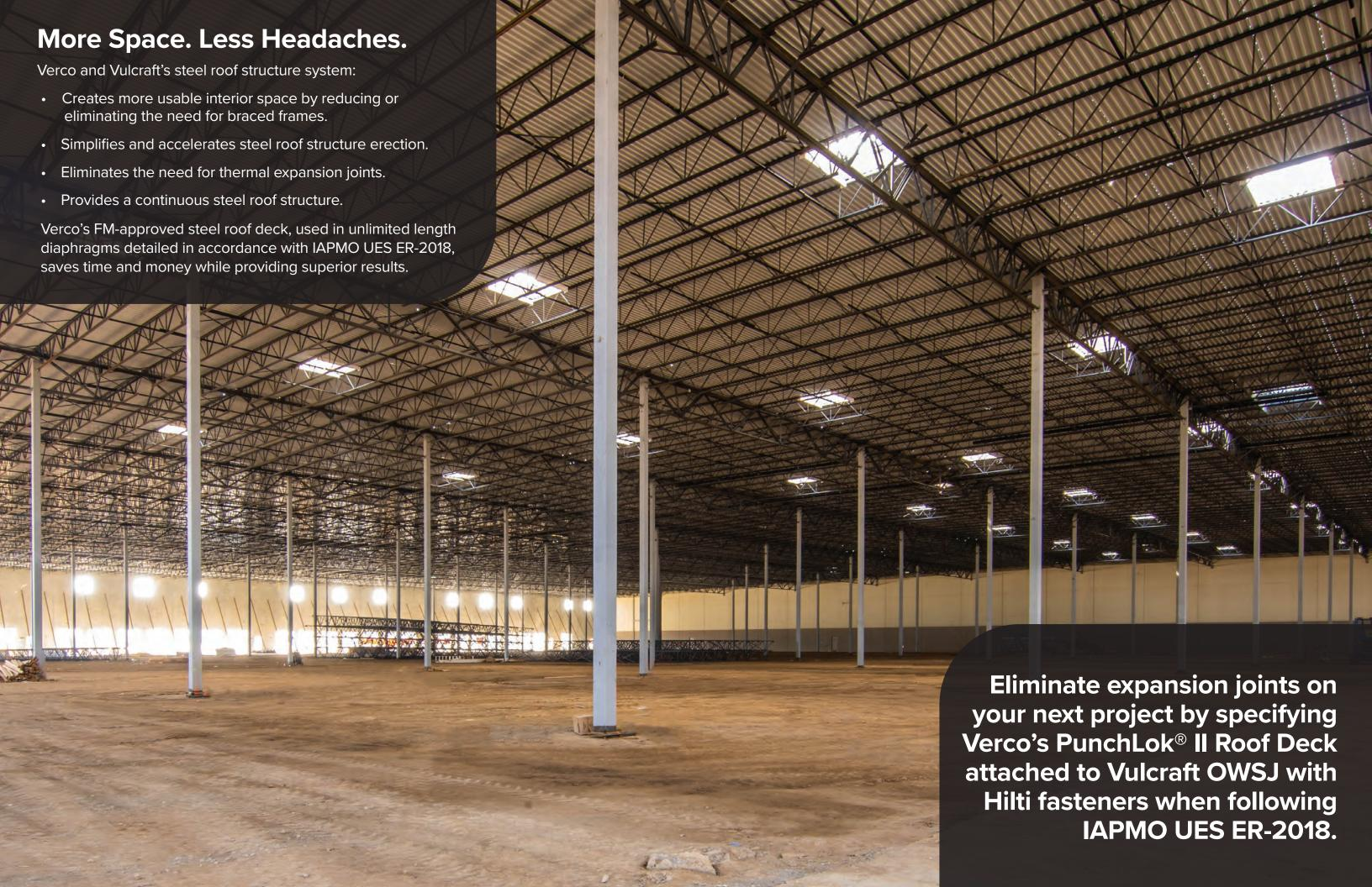
Design roofs free from steel deck thermal expansion joints through the inherent ductility of the patent pending, IAPMO UES ER-2018 recognized, Verco diaphragm system using the PunchLok® II System attached to Vulcraft OWSJ with Hilti PAFs.
